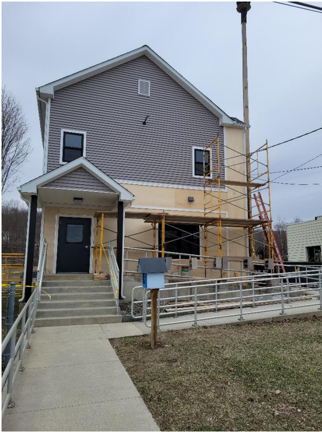
Getting ready to finish the front.
